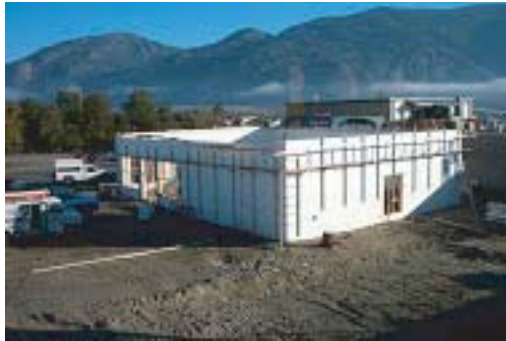
Main walls to roofline
