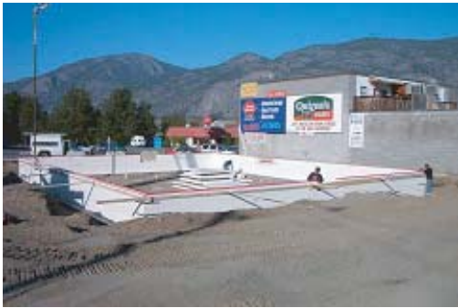
Frost wall up and poured in three hours
